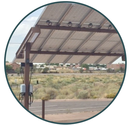
Solar panel equipped charging station A solar powered EV charging station at New Mexico's Petroglyph National Monument.
